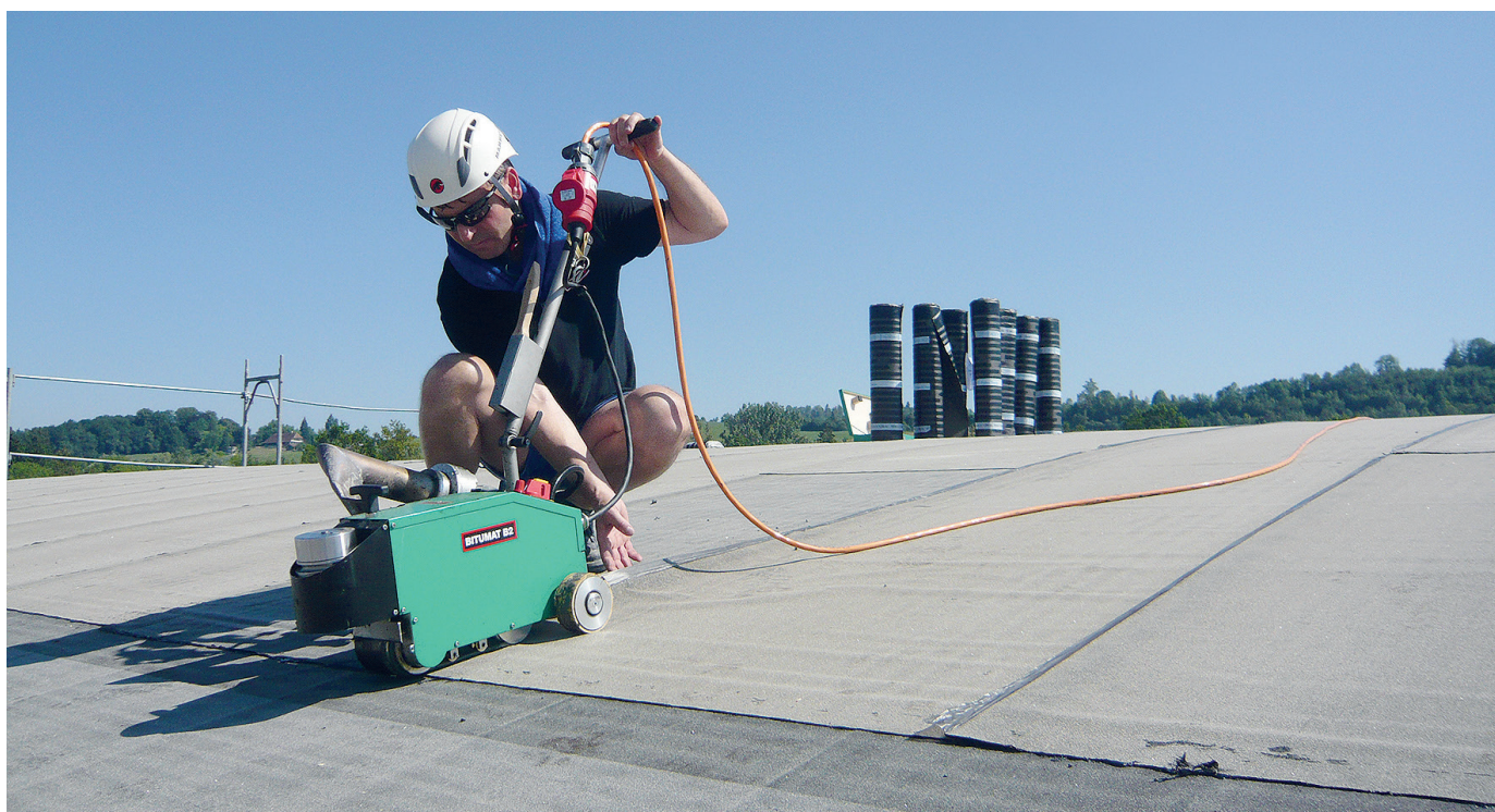
Welding modified bitumen with hot air, thus eliminating open flame.
