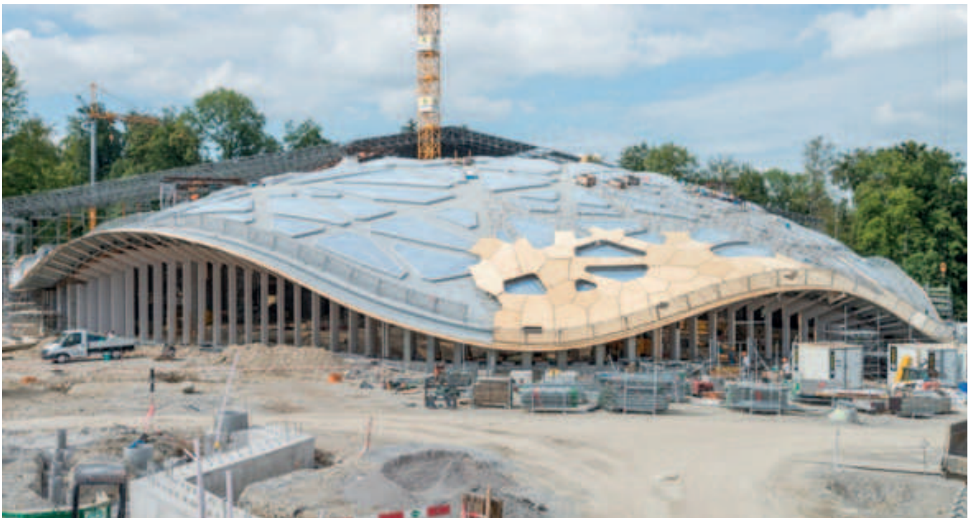
Elephant park at Zürich zoo, reliably sealed with a thermoplastic membrane.
