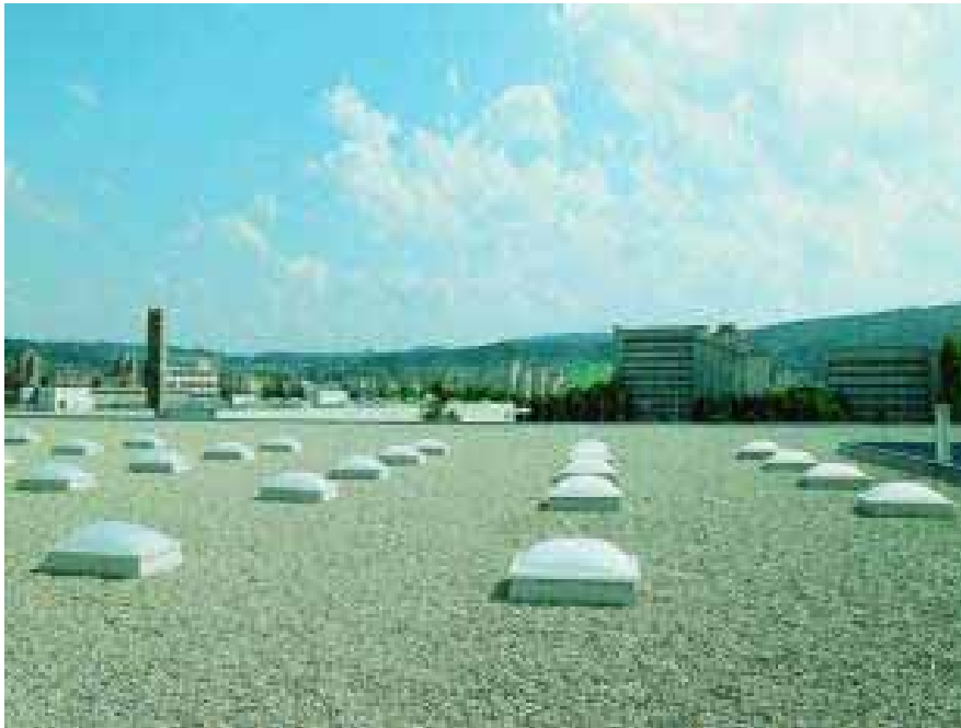
PVC flat roof gravel ballasted
