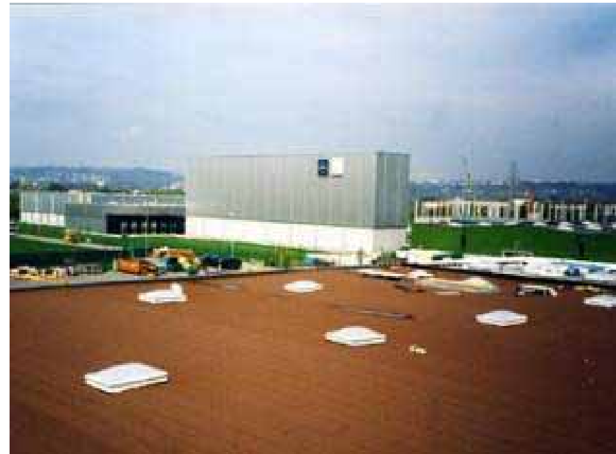
Bitumen flat roof mechanically attached
