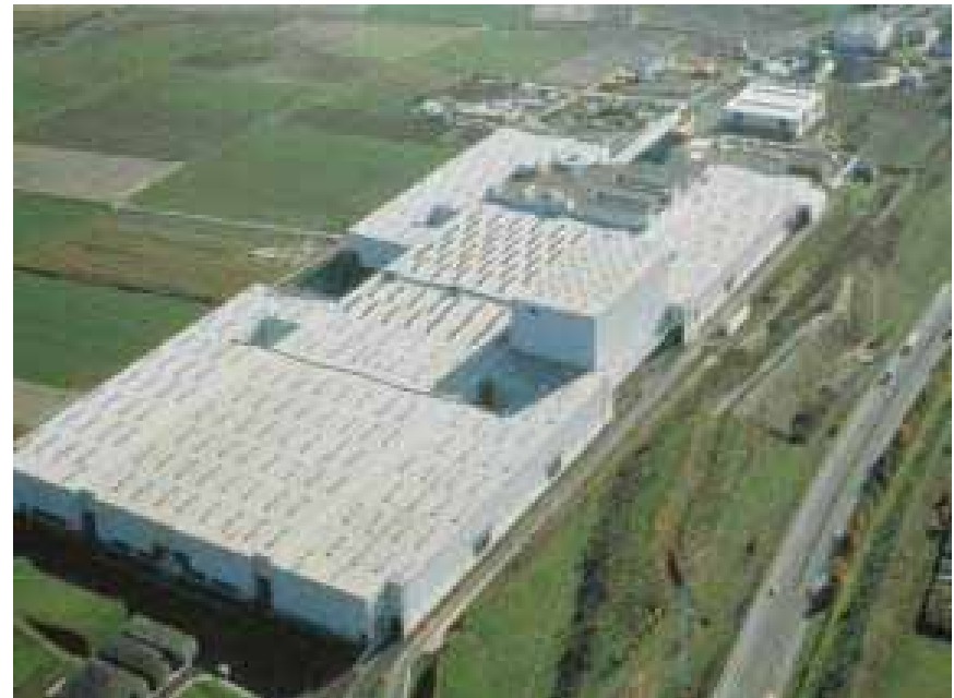
TPO flat roof mechanically attached
