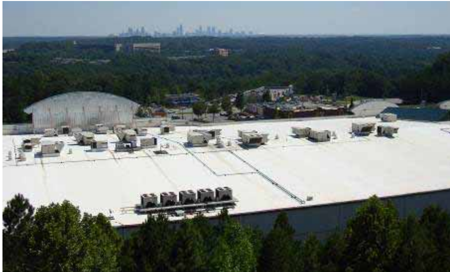
PVC flat roof mechanically attached
