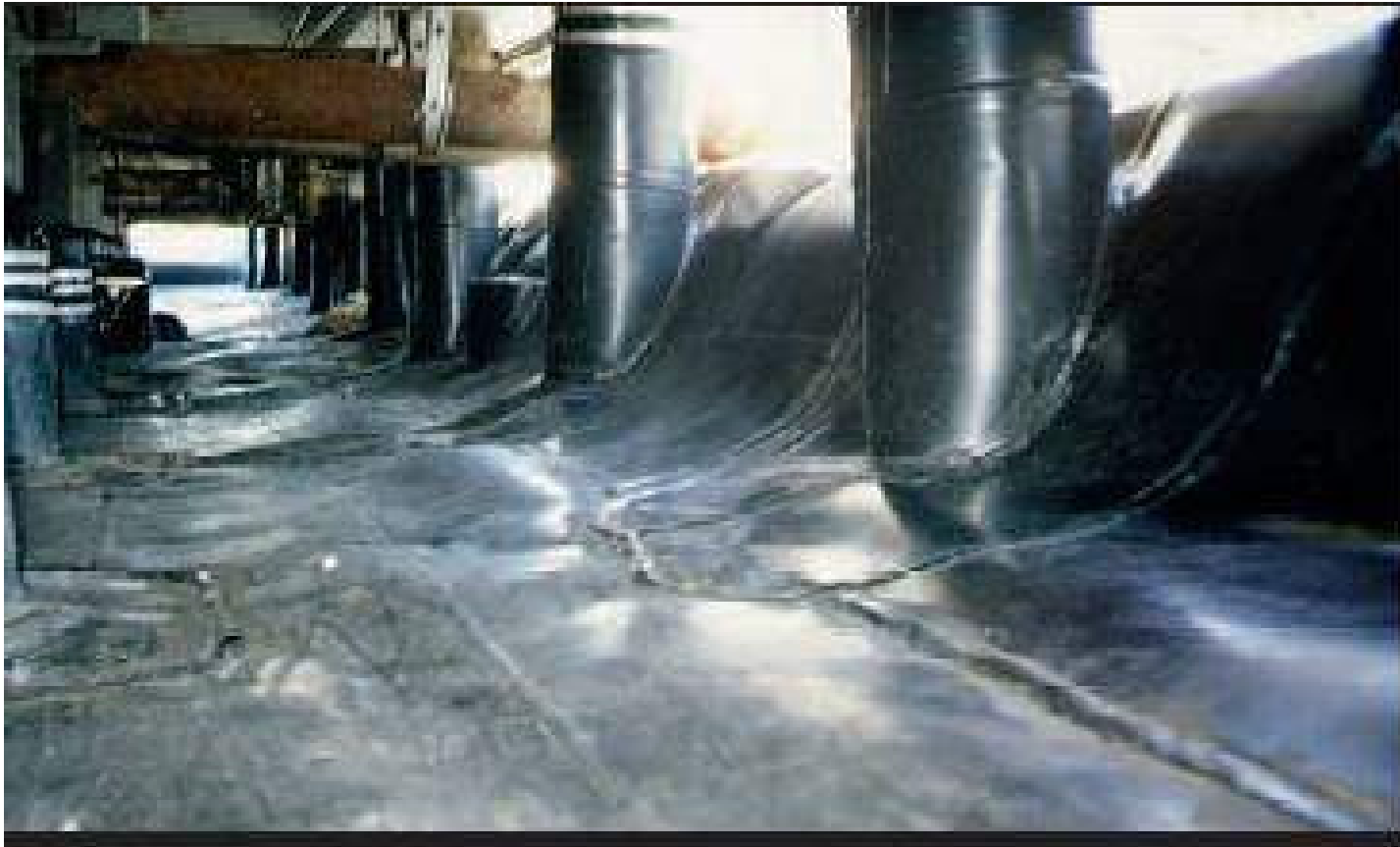
Secondary containment for ground water protection
